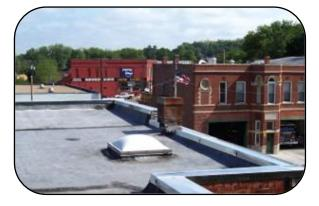
Fire Retardant (FR) EPDM membranes are specially formulated to inhibit spread of flame and meet or exceed code body testing criteria for fire retardant roofing membranes.
