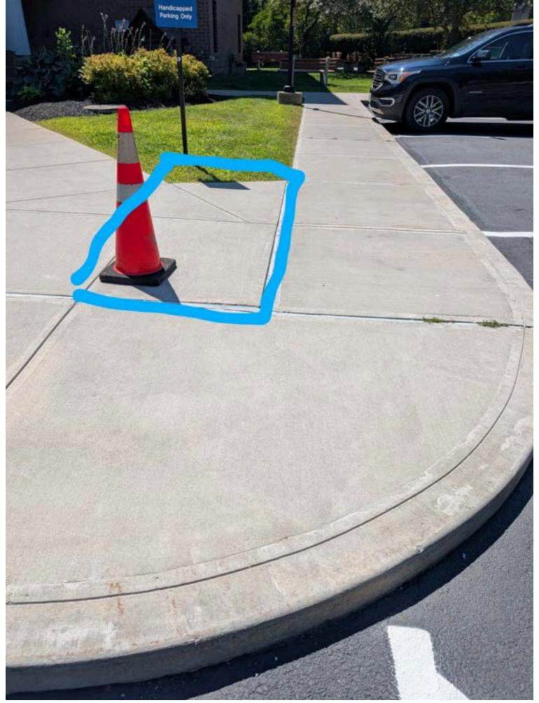
We recommend that the concrete in the blue rectangle in the photo above be removed and replaced. The second option is grinding down the trip hazards, but aesthetically this is less appealing, although it may be
